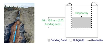
The SAAX is installed inside a 50mm diameter plastic pipe and placed in a shallow (300mm-500mm) trench, backfilled with sand.
